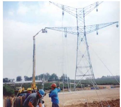
Controlled cable tensioning
